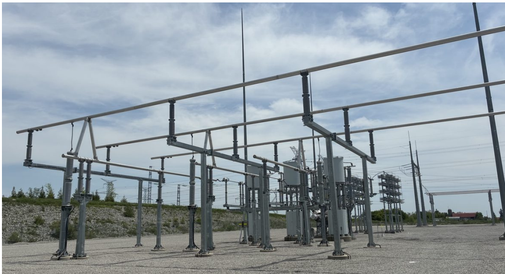
Existing plant being relocated
